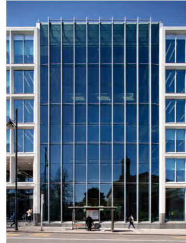
The Lambeth Civic Centre in London is BREEAM Excellent certified.
