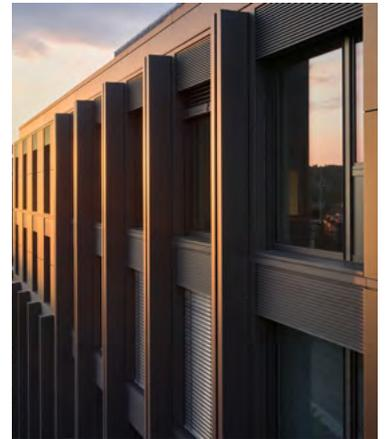
Seven storey office building in new wood-concrete hybrid construction with mixed use of office space, medical practices and other services. The cladding material of the energy efficiency house is a solar façade made out of bronze SKALA modules.
