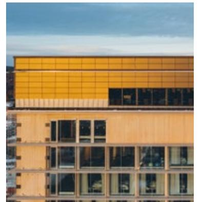
This new multi-purpose building was constructed entirely of wood. Our bronze-colored SKALA modules enclose the SPA area located on the top floor at a height of 80 m and are a wonderful addition to the wooden construction of the building.
